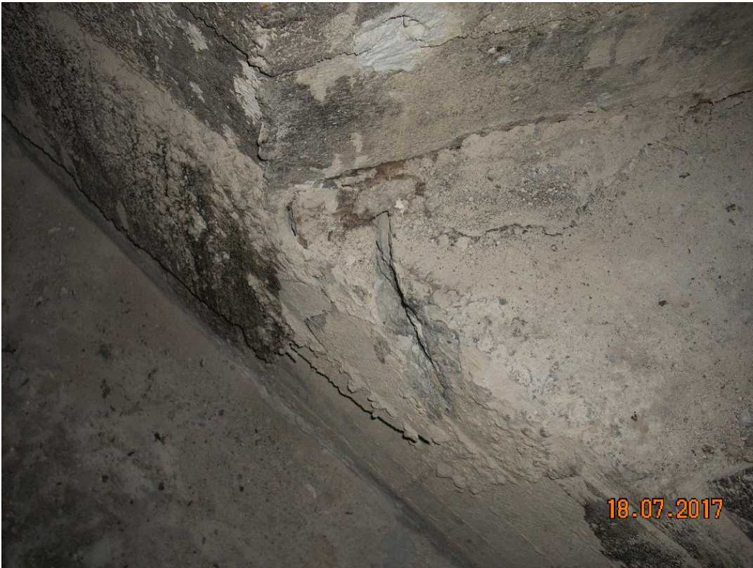
Fig. 2-31: Photo of the damaged deviator
