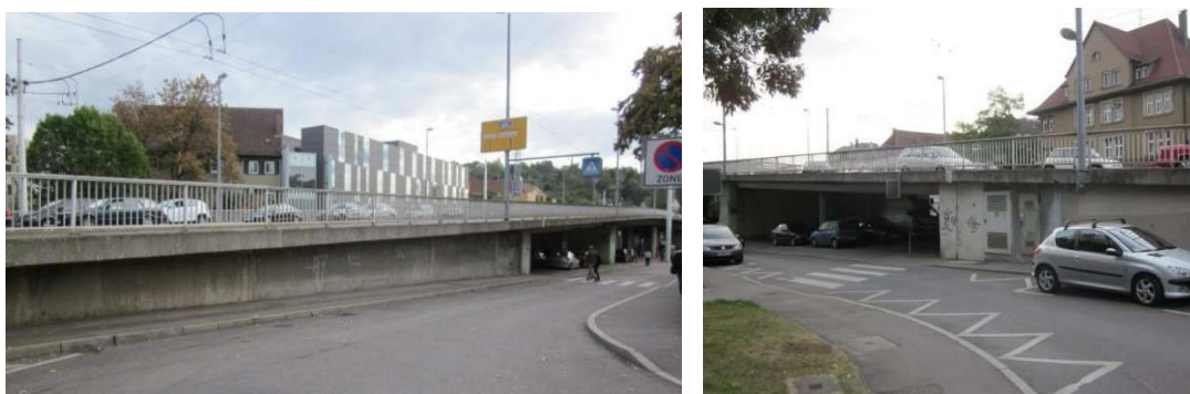
Fig. 3-11: View on two-span bridge form both sides showing good accessibility from underneath
