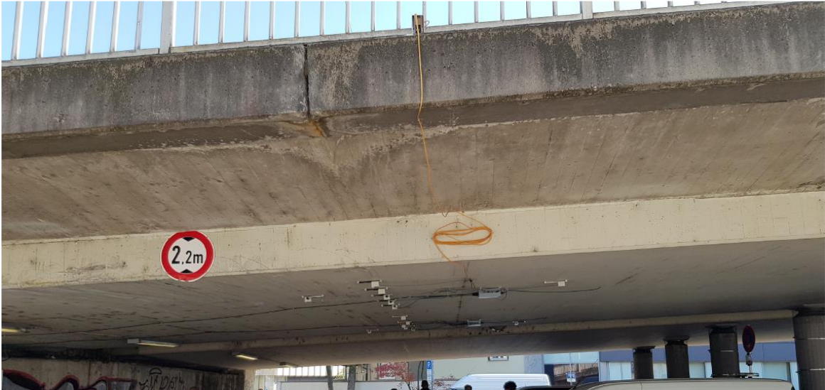
Fig. 3-1: View of the installed sensors
